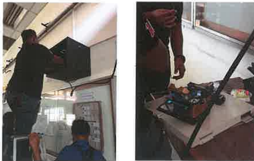
Figure 3.6: splicing and install it in the rack
