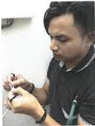
Photo 5: termination UTP cable, using type b
