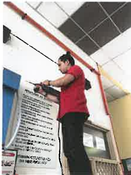
Figure 3.5 : drill for installing AP(Access Point)
