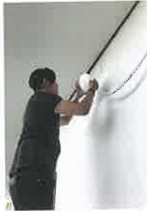
Photo 6: mounting/ installing AP
