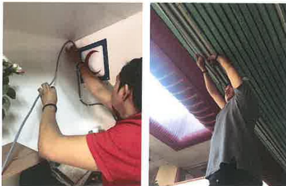
Figure 3.4: setup routing for fiber optic and power cable
